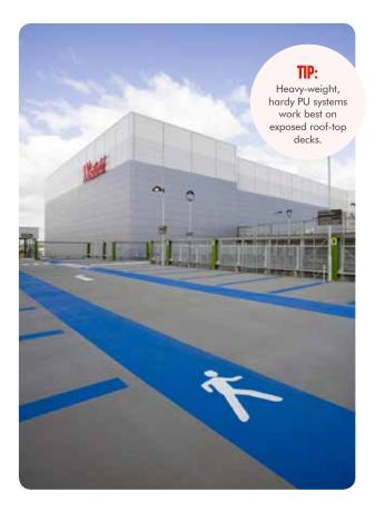
Highly resistant polyurethane resin-based deck coatings can be used to prevent the early onset of corrosion, providing a protective barrier between the contaminants and the host substrate.
